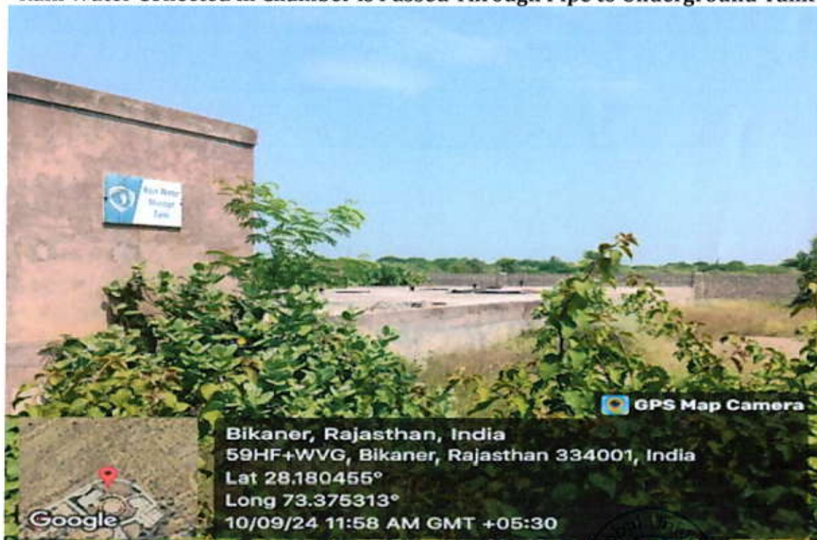
Underground Tank for Storing Rain Water
