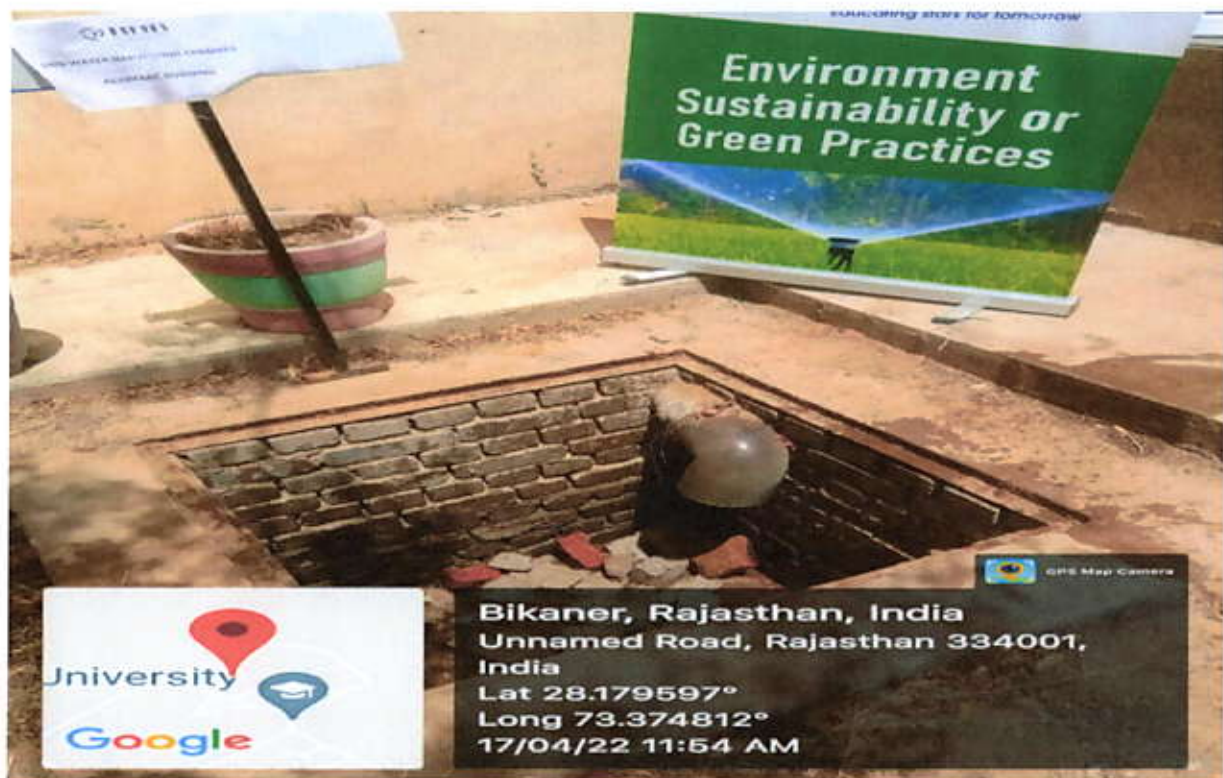
Recharge Chamber through which Rain Water is diverted to Storage Tank
